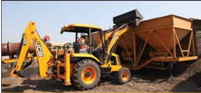
Hopper feeding for ready mix concrete
