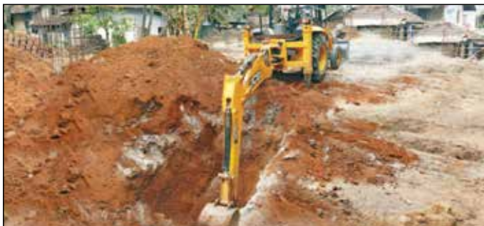
Rural infrastructure & square hole
