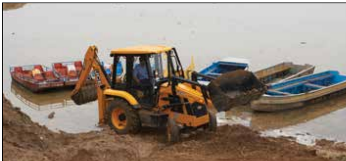
Cleaning of sewages
