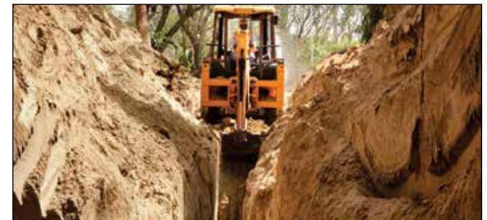
Trenching & pipe laying
