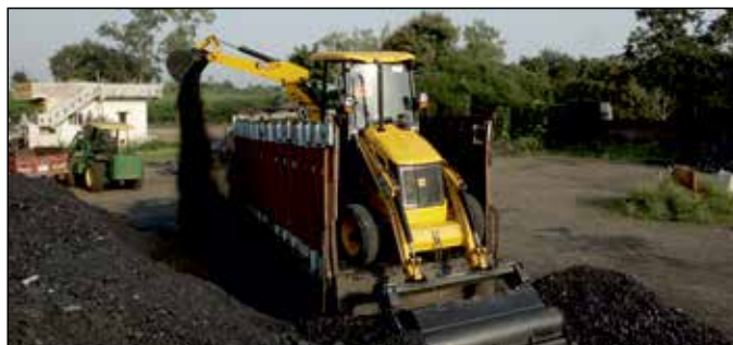
Coal & limestone factory loading / unloading
